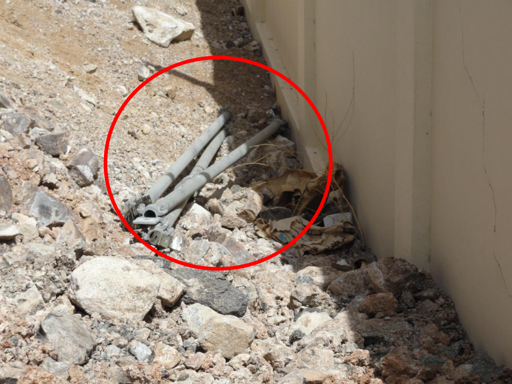
Dismantled 33 KV Busbars Tubes
