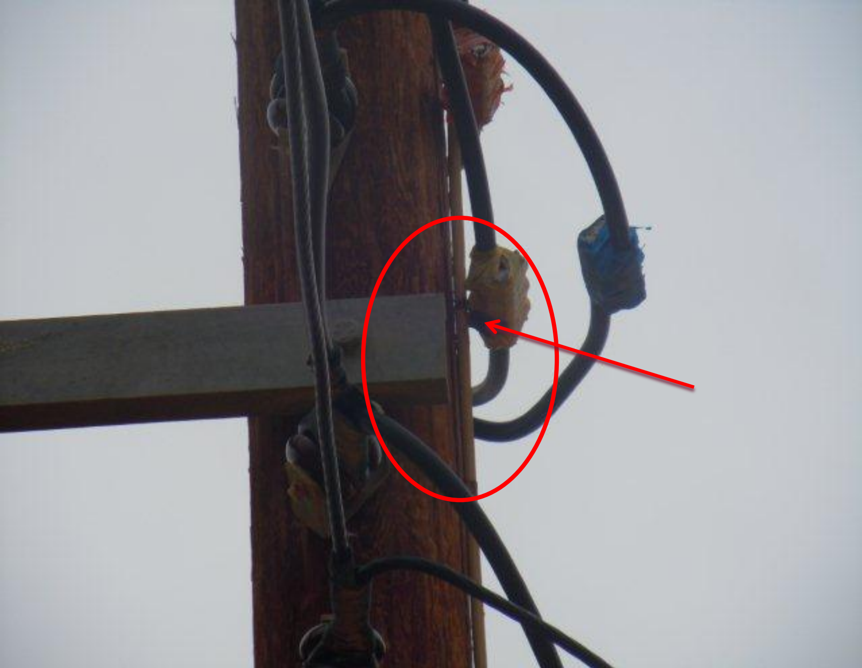
Point of Electrical Leakage Current
