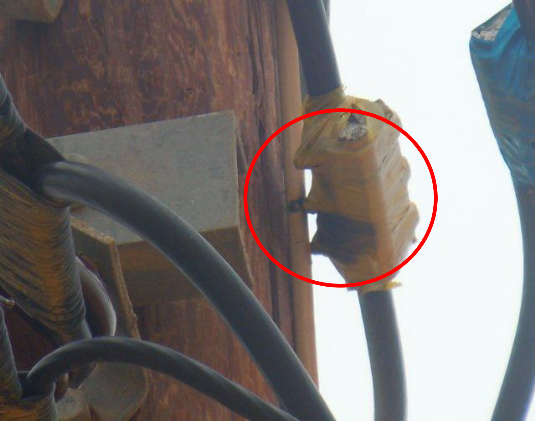
Point Of electrical Flashover
